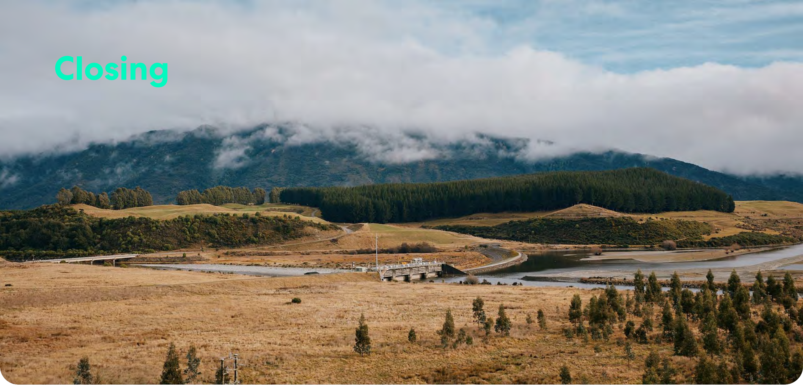
Manapōuri Lake Control structure, Fiordland.
