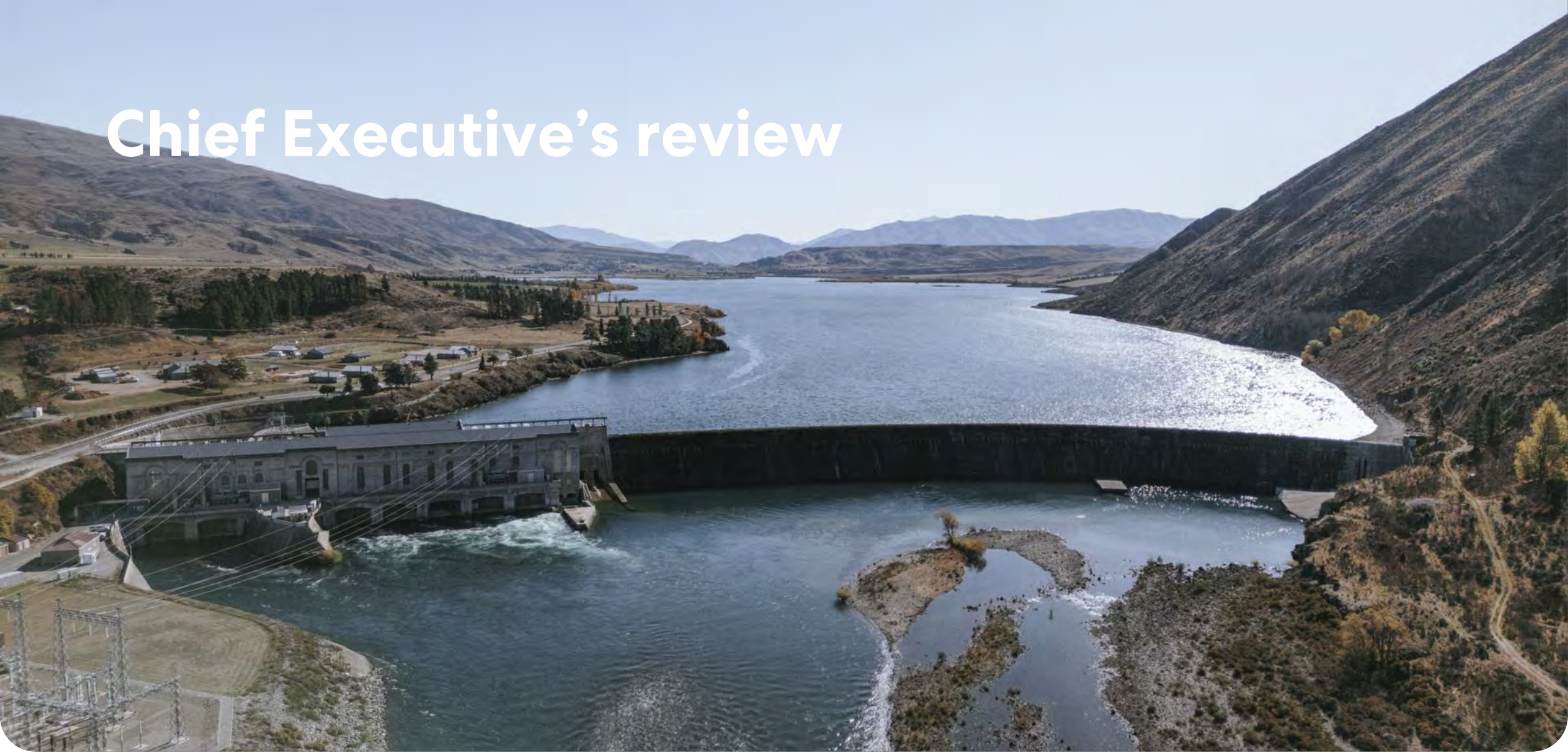
Waitaki Power Station in South Canterbury.
