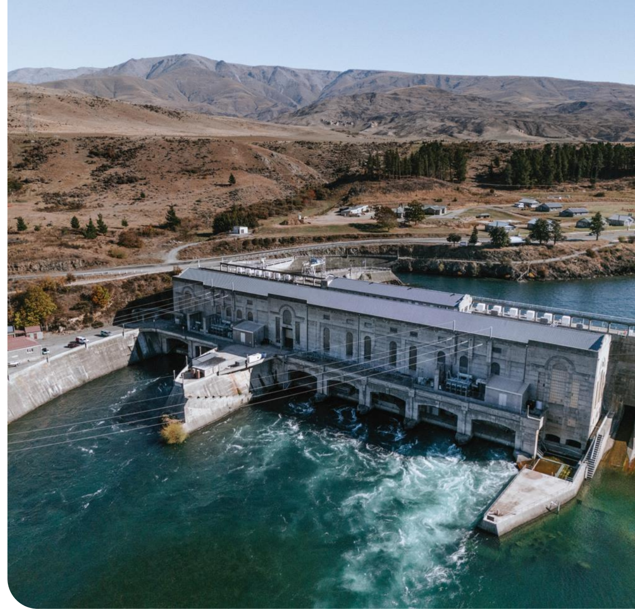
Construction of the Waitaki hydro power station originally began in the 1930's.
