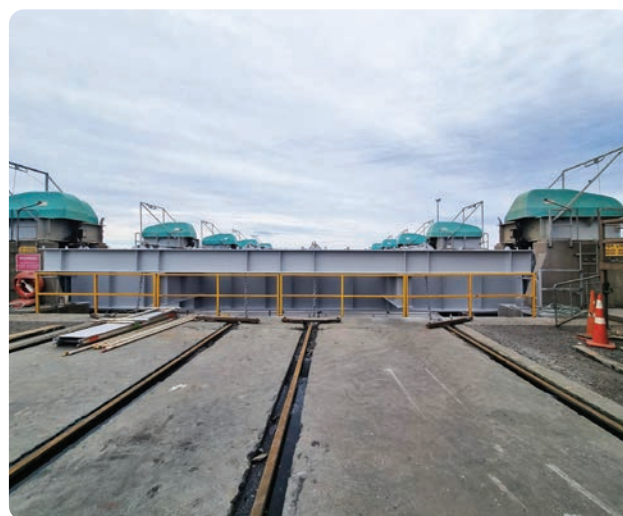
Stage 2 of the Syncrolift structural steel refurbishment.
