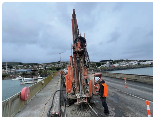
The bridge to the Island Harbour undergoing a seismic performance trial.
