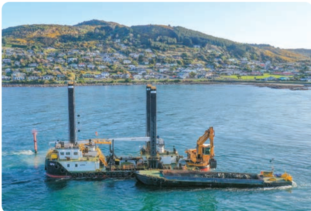
2022: Removal of already fractured and fragmented rock from drilling and blasting that took place in the 1970s and 1980s was the first step in deepening the channel.
