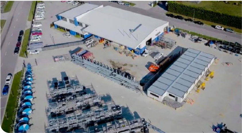
PGW Water Branch in Rangiora, North Canterbury.
