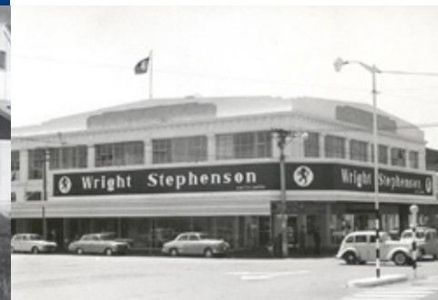
Wright, Stephenson & Co Ltd Blenheim branch. Department Store, 1966. Image credit: Fletcher Trust Archives P4004/13.
