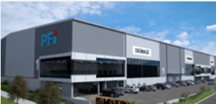
FUTURE DEVELOPMENT - STAGE 1 UNDER CONSTRUCTION
