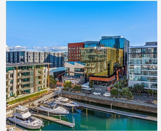
FY23: Wynyard Stage 3 development undertaken in PPILP
