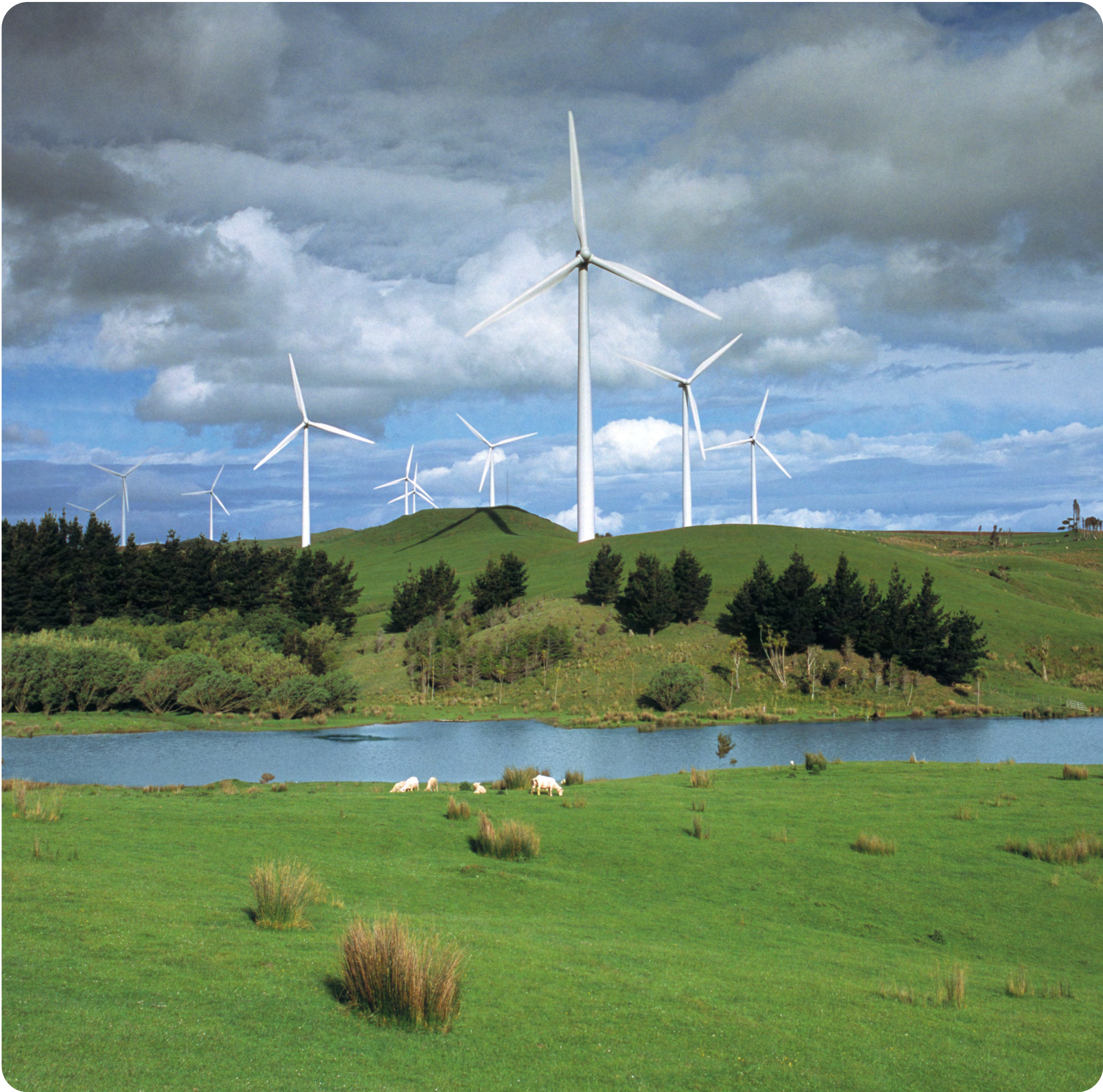
ABOVE: Te Āpiti Wind Farm.
