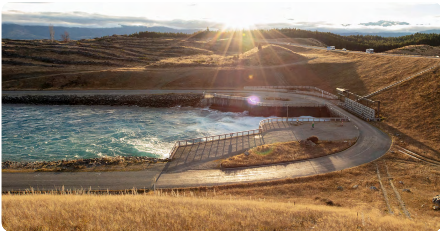
ABOVE: Water from Lake Pūkaki flowing through the Pūkaki Canal inlet (Gate 18) and into the Pūkaki Canal.
