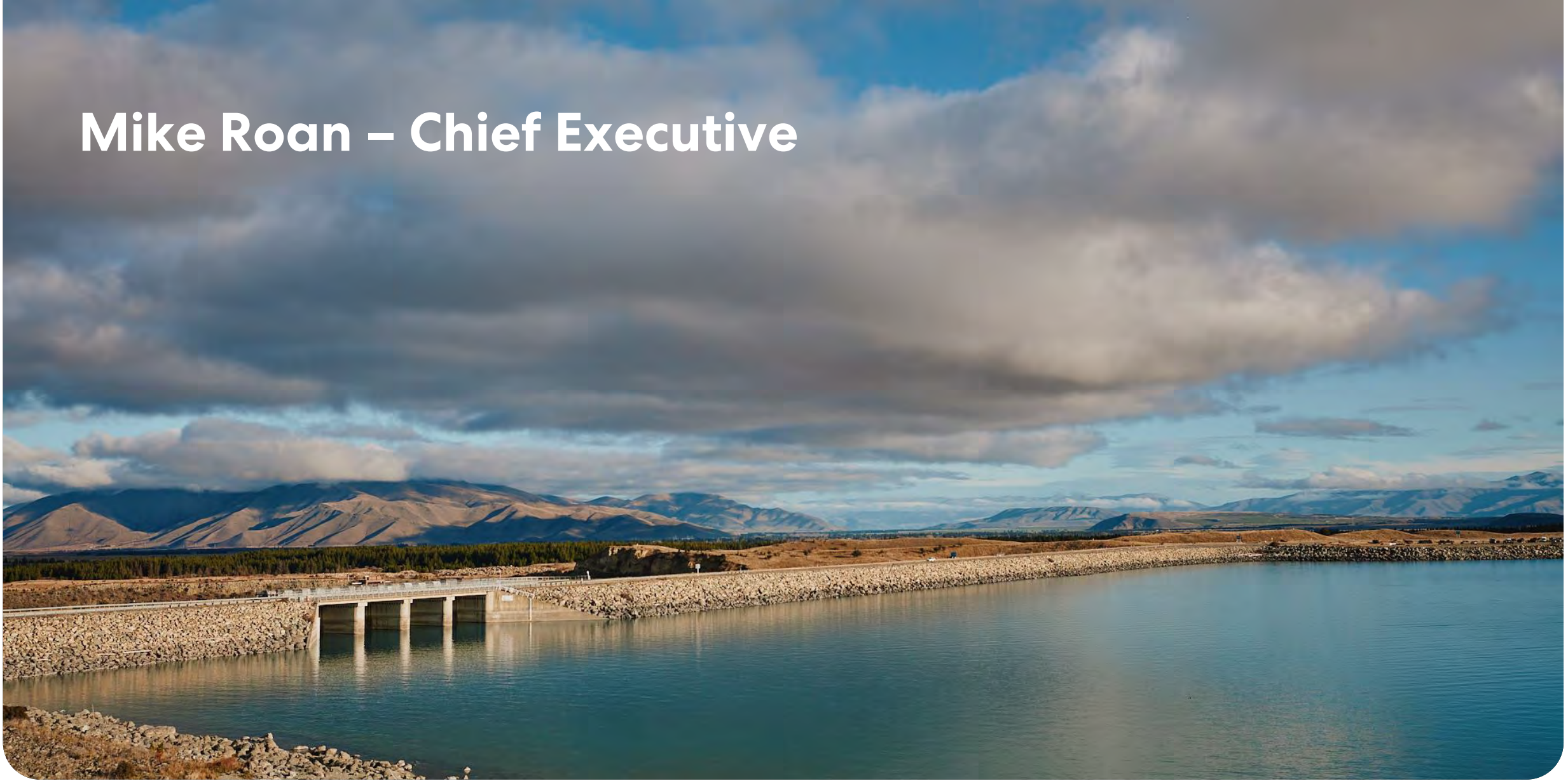
Control structure and spillway, Lake Pūkaki
