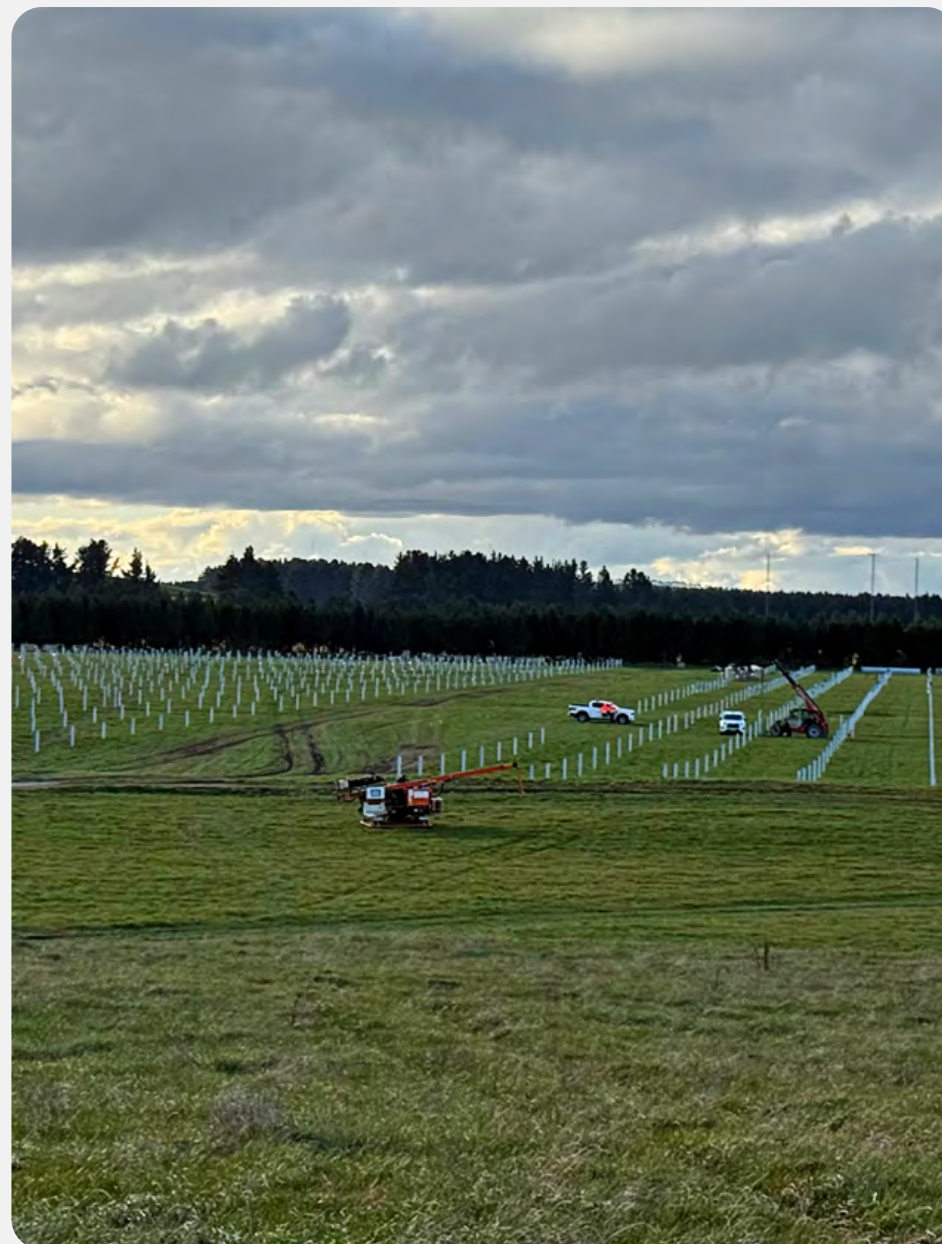
ABOVE: Te Rahui Solar Farm under construction.
