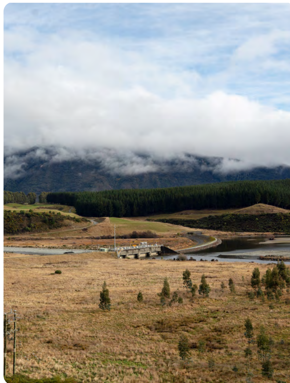
ABOVE: Manapōuri Lake Control Structure, Mararoa Weir.
