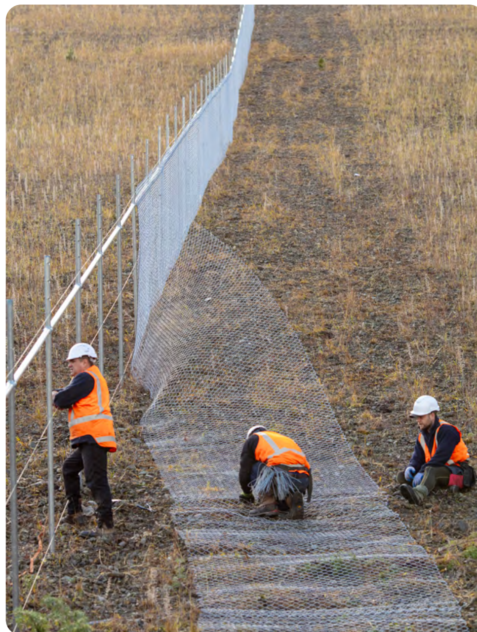
ABOVE: Fencing installation Benmore Power Station, Ōtematata.
