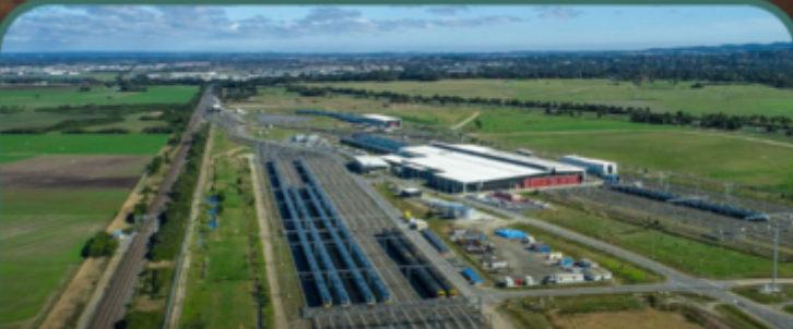
Our rail maintenance depot in Pakenham East, VIC supporting population growth
