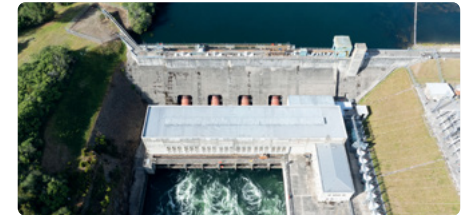
Committed to next phase of hydro refurbishment programme.
