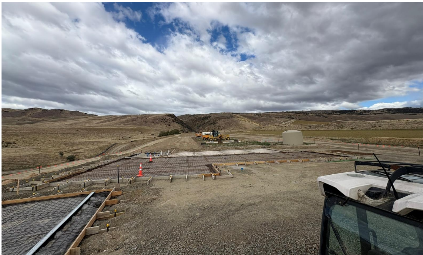
Figure 5. Administration building pads - at debouchment of Shepherds Valley mine entrance
