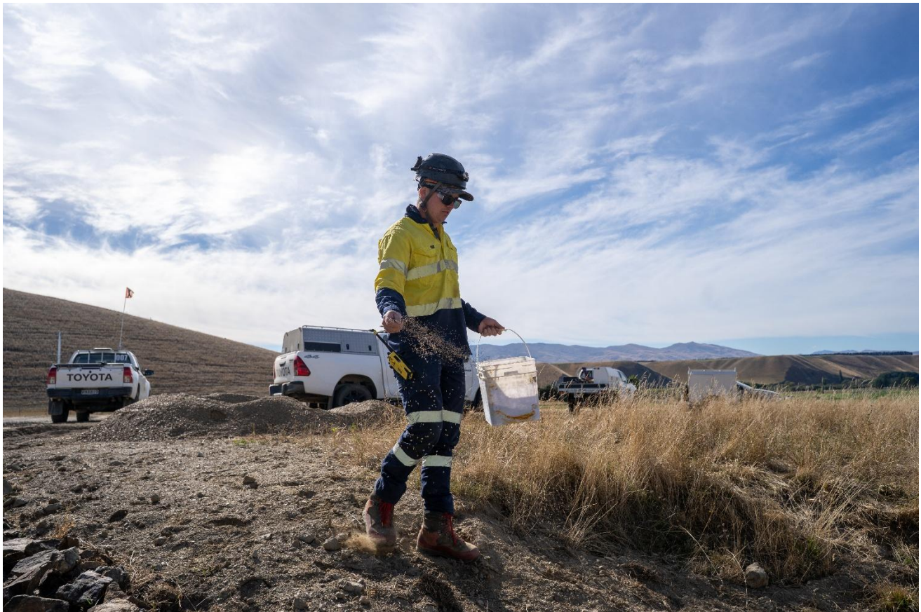
Figure 4. Reseeding backfilled trenches for immediate rehabilitation of disturbed areas
