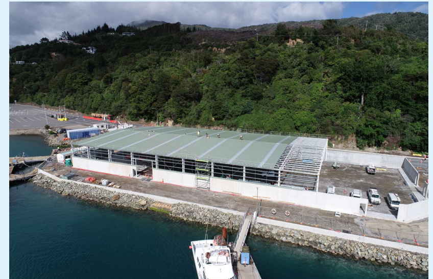
Build of Westshore Warehouse in Picton underway
