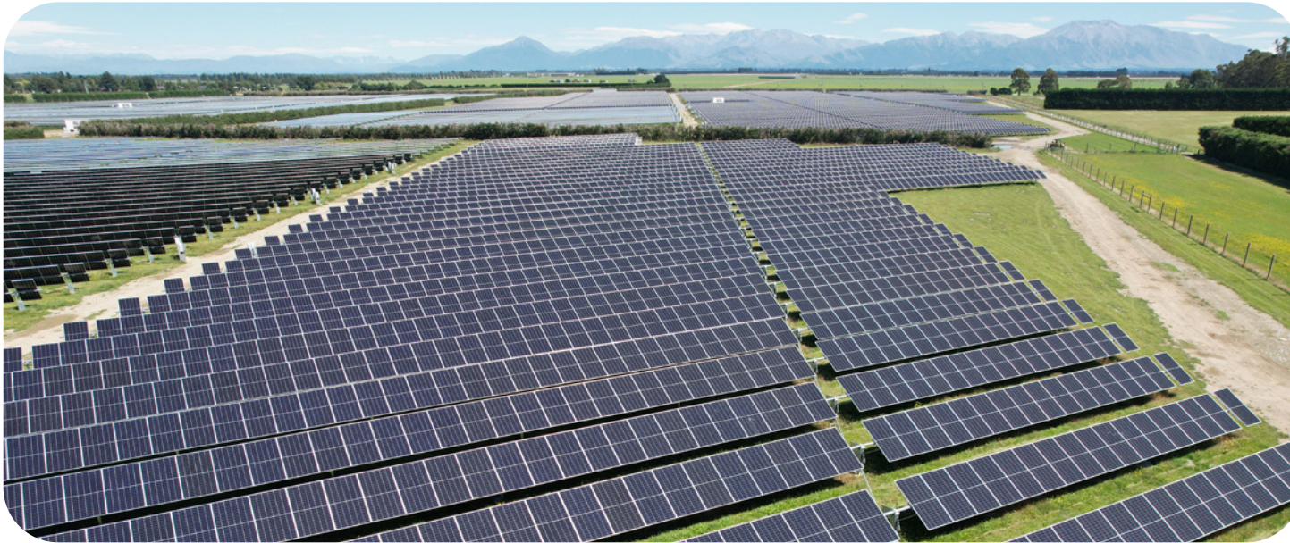
Lauriston solar farm
