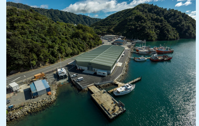
The Westshore Warehouse at Port Marlborough in Picton, serving as a feed storage facility for NZK.
