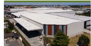
244 Puhinui Road, Manukau
