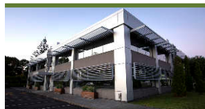
80-120 Favona Road, Mangere
