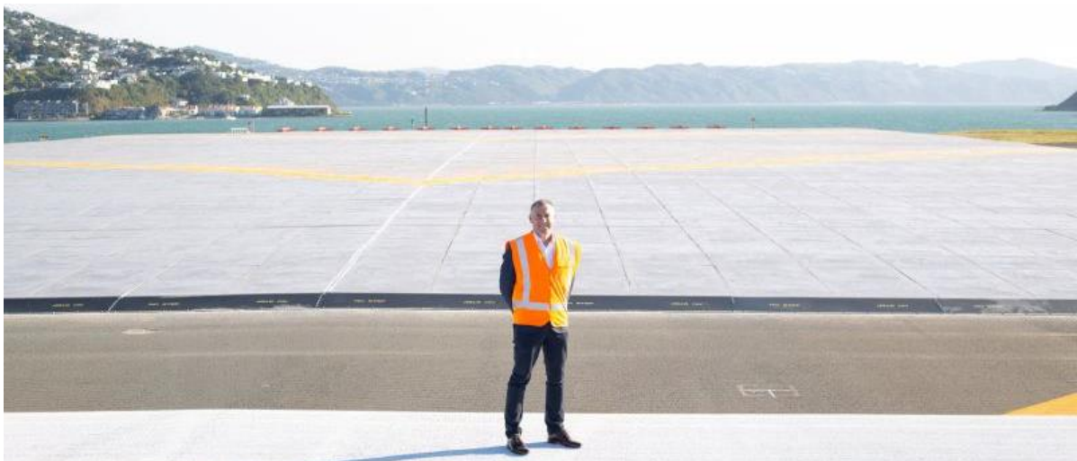
Wellington Airport CEO Matt Clarke in front of the completed northern safety area.
