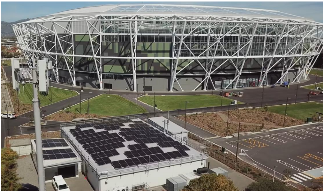
The data centre and mobile tower (foreground) adjacent to the new stadium.
